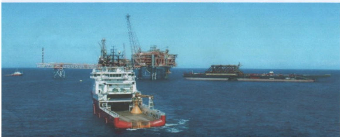
After 4 years of preparations the 24.250 ton NRB deck was installed onto the jacket in just over 6 hours by means of the float-over method. This will be the largest to date open water float-over done and a huge achievement by the crew and projecteam of the H-851 . Accompanying tugs were the DEEP SEA 1 (28.000 HP) seen in the picture and the MAERSK PROMOTER, FAR GRIP and LEWEK SWAN . Many thanks to the projecteam and crew of the H-851 Photo : Willem van Woercom (c)
