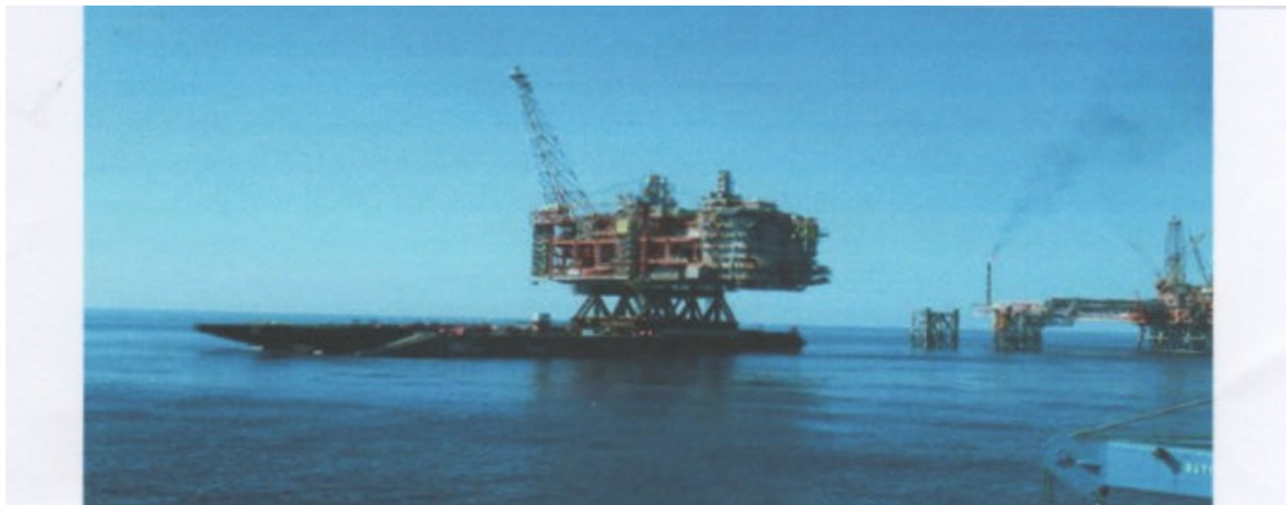
After 4 years of preparations the 24.250 ton NRB deck was installed onto the jacket in just over 6 hours by means of the float-over method. This will be the largest to date open water float-over done and a huge achievement by the crew and projecteam of the H-851 . Accompanying tugs were the DEEP SEA 1 (28.000 HP) seen in the picture and the MAERSK PROMOTER, FAR GRIP and LEWEK SWAN . Many thanks to the projecteam and crew of the H-851 Photo : Willem van Woercom (c)
