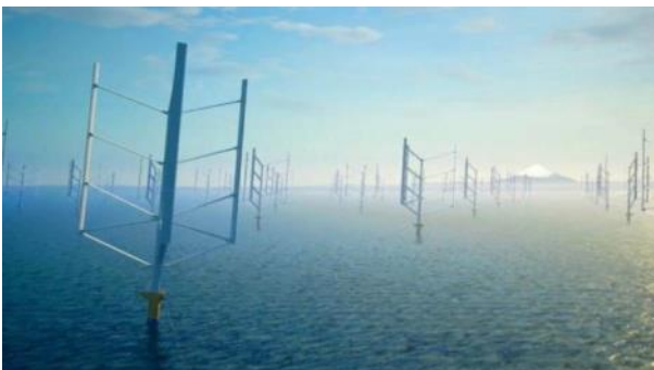
Floating vertical access wind turbines
